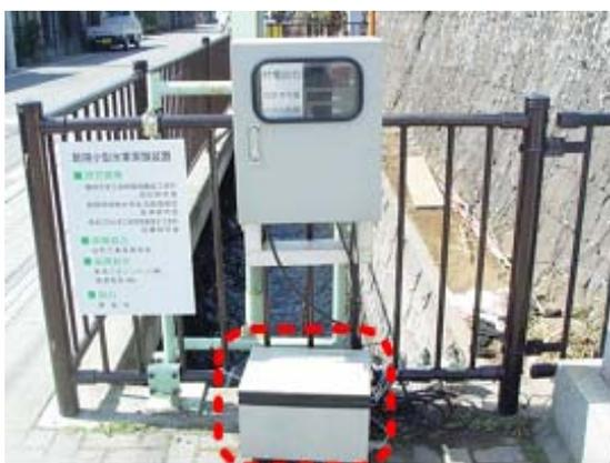
Fig.5 Installation of the power conversion system.
